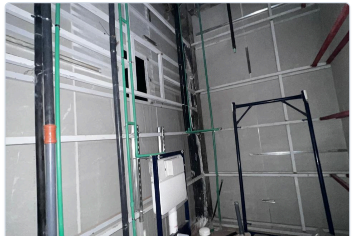
PPR potable water supply and concealed sanitary piping installation
