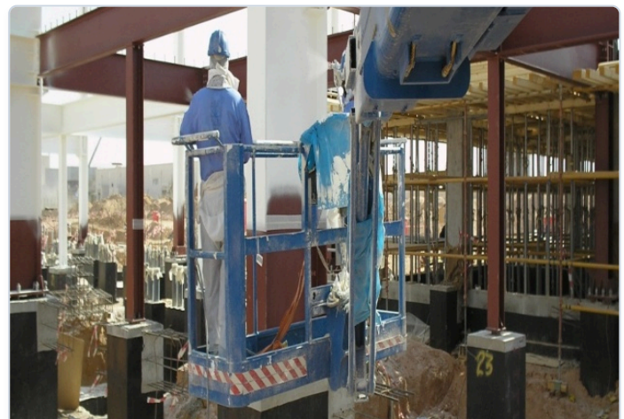
Abrasive blast cleaning to Sa 2.5 standard per ISO 8501
