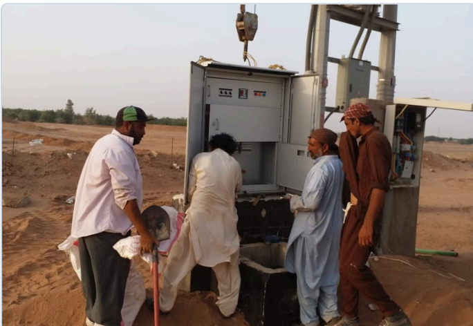
Power cable pulling, dressing, and field electrical panel termination
